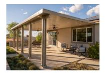
2.9 Balcony Cover: A single story architectural projection located at balcony levels that provides partial weather protection but remains open on three sides. One end of the cover is supported by the building while the opposite end is supported by a post and beam configuration.
